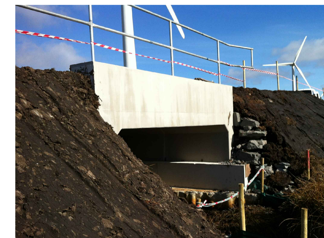
Bottomless Box Culvert Crossing
