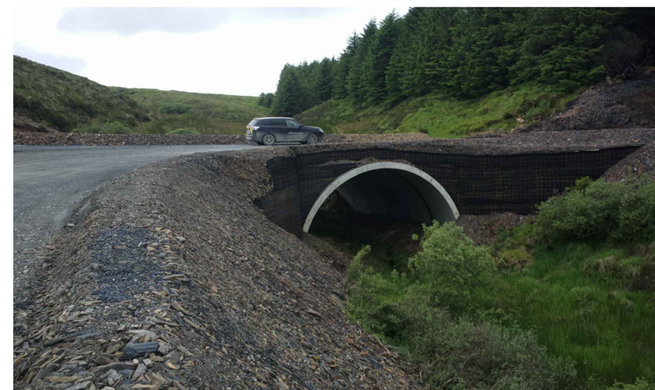
Bottomless Arch Culvert Crossing
